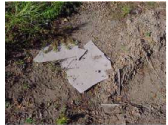
Photo 6 – Fragments of Asbestos Cement sheeting on ground surface
